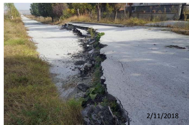
Figure 3. The main E-W trending surface fracture immediately after the landslide (top) and fifteen months later (bottom). It is clear that the fracture is still active and the displacement exceeds 0.7 meters.
